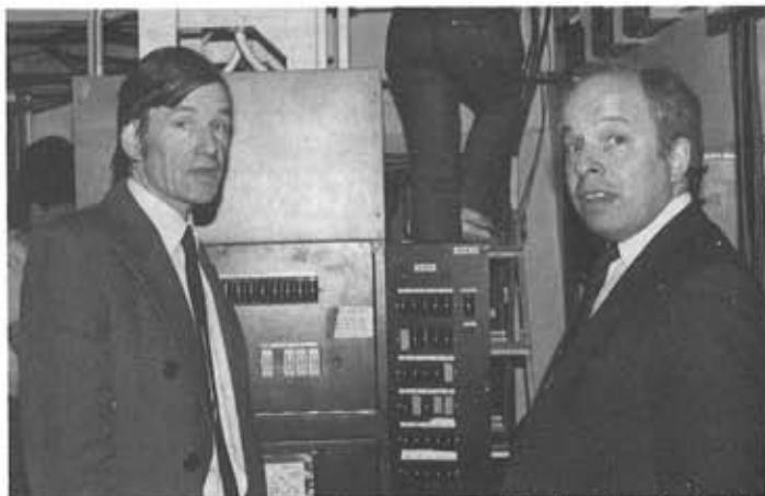
Northern Light's Mike Smith (left) and Roger Fox in discussion during the height of the installation work in mid-January.
